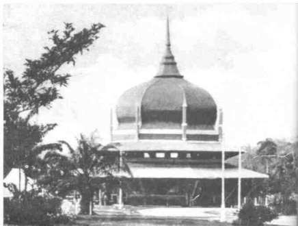
The durbar was held in this octagonally-shaped building, which was specially erected in the Lake Gardens.
